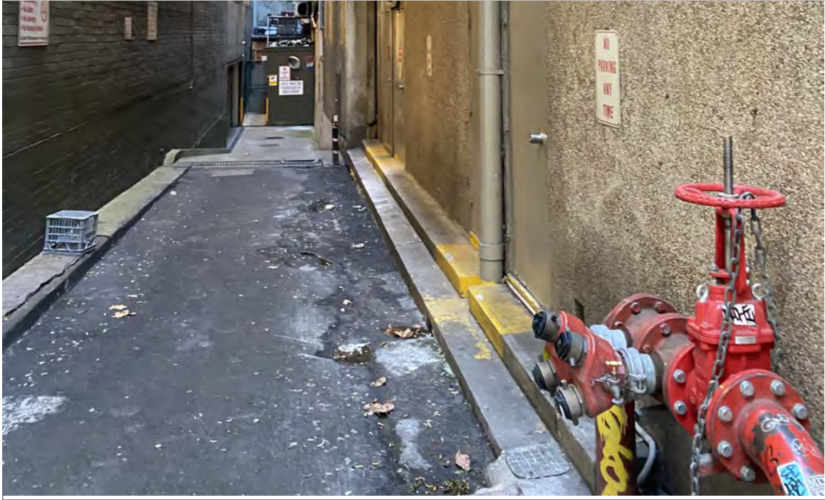
Photo 1: Alleyway along Pitt Street, looking towards the west
